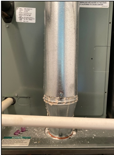
Efflorescence observed on vent pipe at joints.
