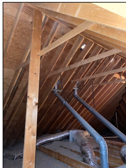
Roof Rafters and Ceiling Joists
