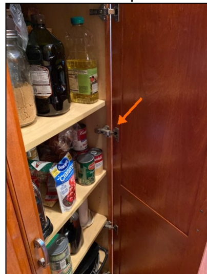
Cabinet doors have broken/loose hinges.
