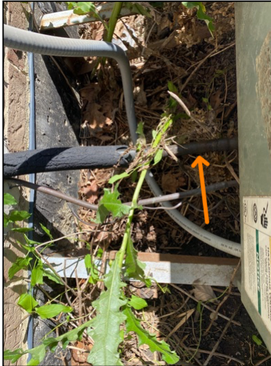
Missing insulation at A/C unit.
