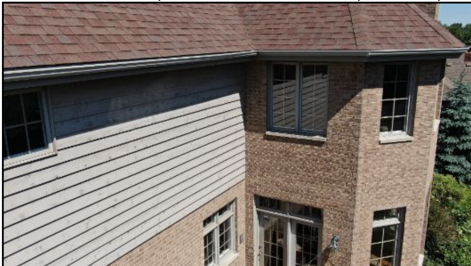
Deteriorated paint on the exterior should be repaired and painted.
