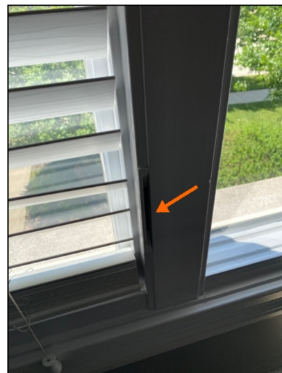
Lock/Latch is Broken/Missing.
