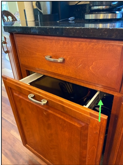
Broken drawer guides noted. Recommend having a qualified contractor replace the guides.
