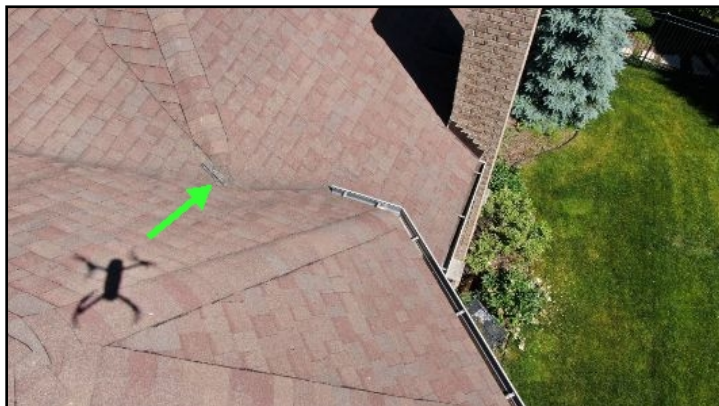
Some shingles damaged.
