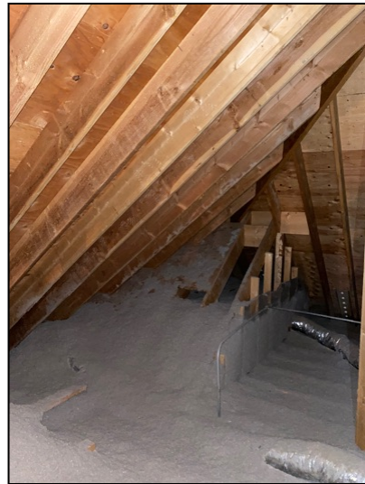
Roof Rafters and Ceiling Joists
