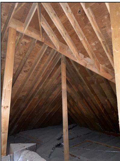
Roof Rafters and Ceiling Joists
