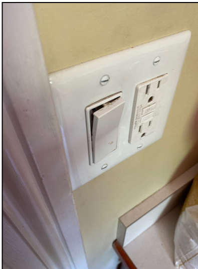
Outlet/Switch is damaged.
