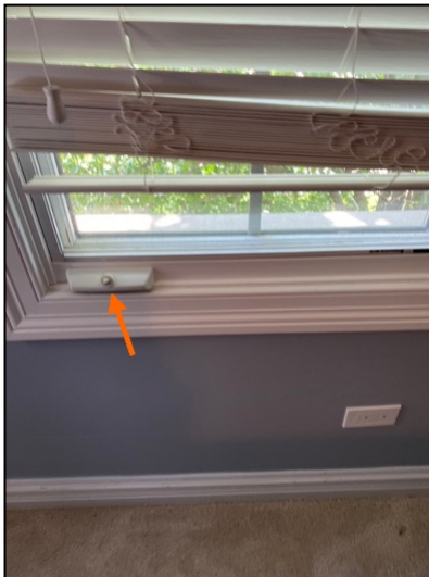
Window(s) not able to open during the inspection. Handle is missing.
