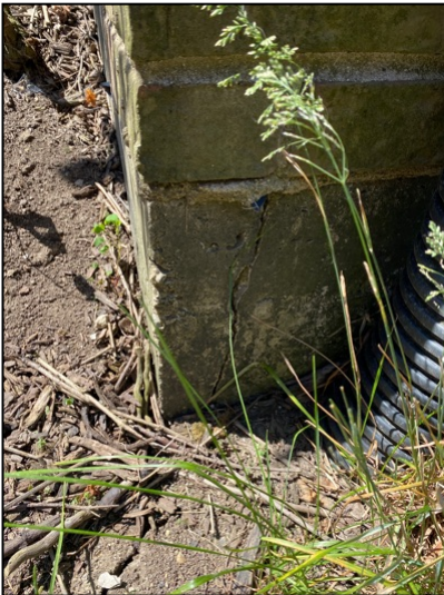
Wedge crack on foundation.
