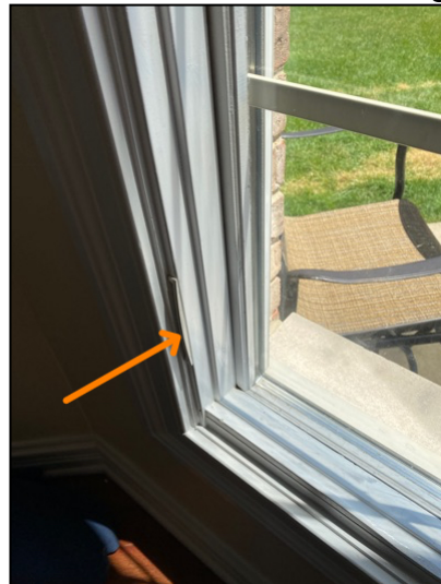
Lock/Latch is Broken/Missing.
