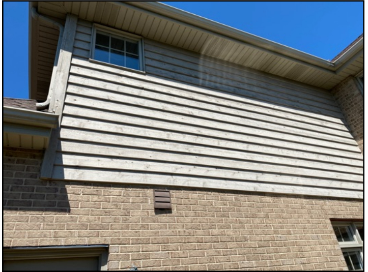
Deteriorated paint on the exterior should be repaired and painted.
