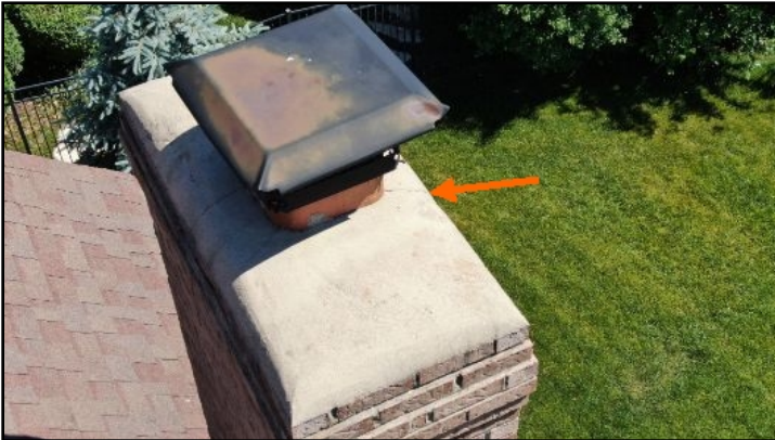
Masonry chimney cap is cracked
