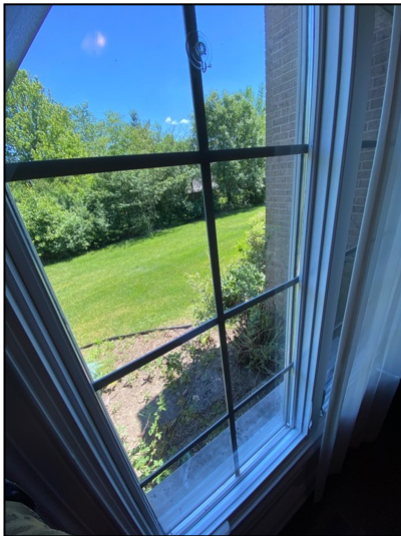
Missing / Damaged screens observed.
