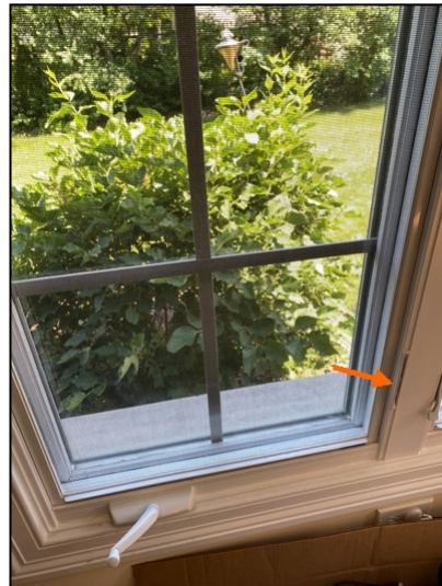
Lock/Latch is Broken/Missing.
