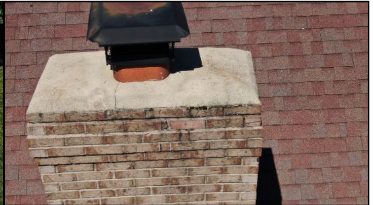
Masonry chimney cap is cracked
