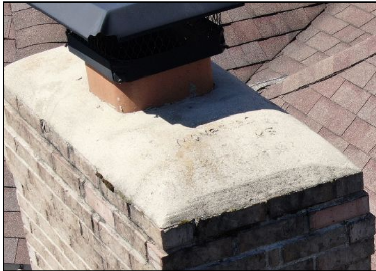
Masonry chimney cap is cracked (and signed and dated).
