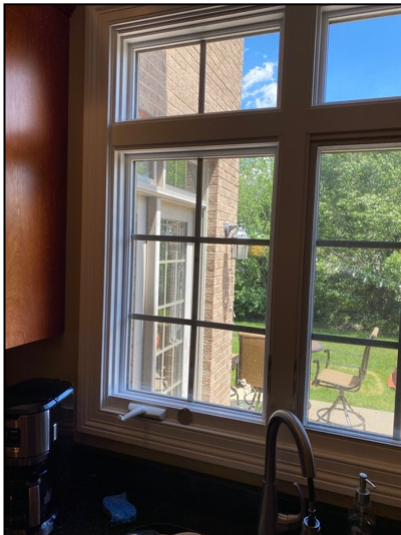
Missing / Damaged screens observed.
