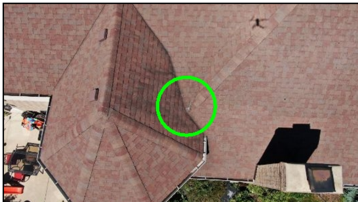
Some shingles damaged.
