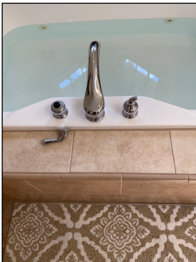
Faucet controls are damaged/broken.
