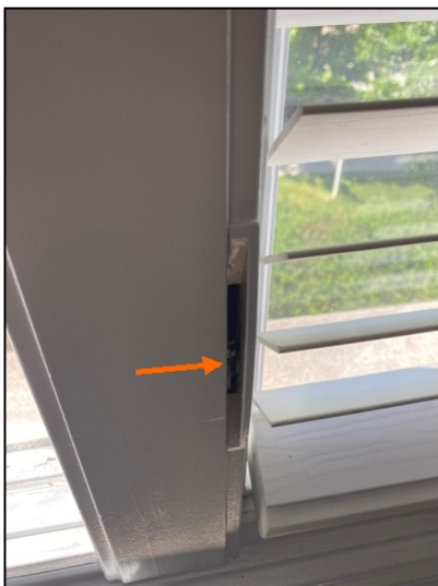
Lock/Latch is Broken/Missing.
