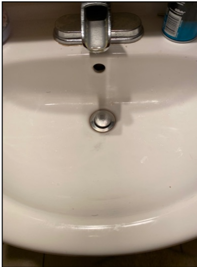
Drain stopper is missing/inoperable.
