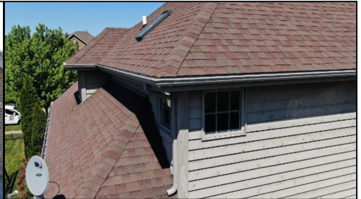
Deteriorated paint on the exterior should be repaired and painted.
