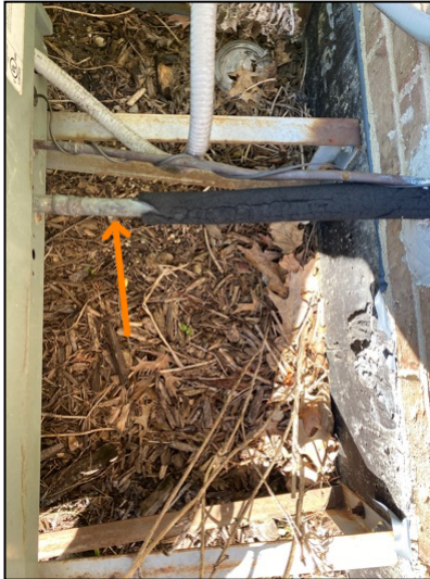
Missing insulation at A/C unit.
