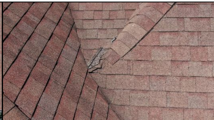
Some shingles damaged.
