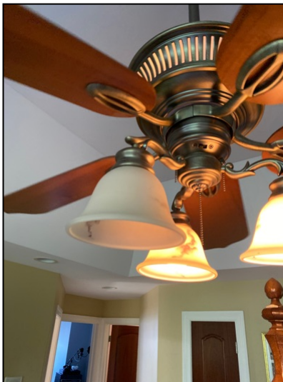
The LIGHT portion of the Paddle Fan did NOT operate at the time of the inspection.
