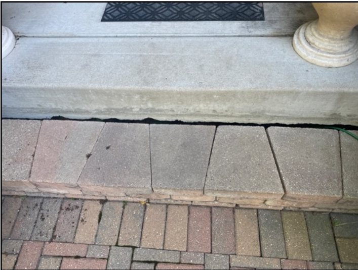
Front brick paver step has settled.
