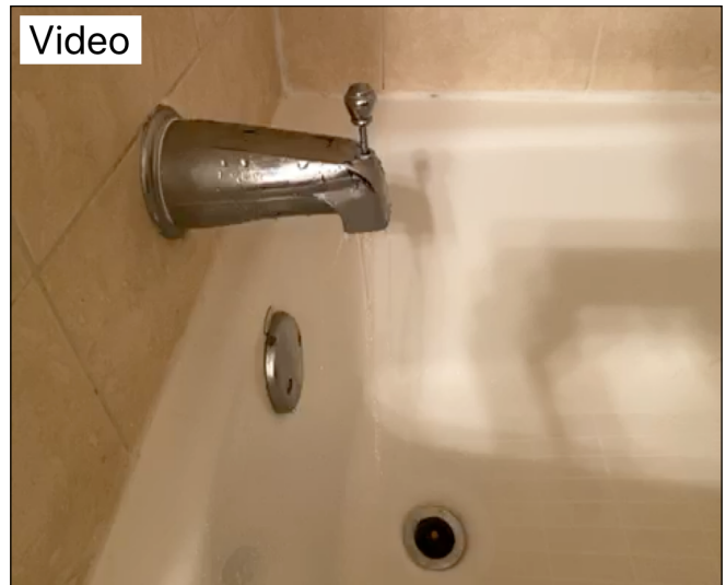
Shower diverter did not operate properly.
