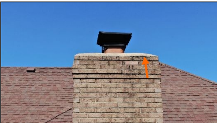
Masonry chimney cap is cracked
