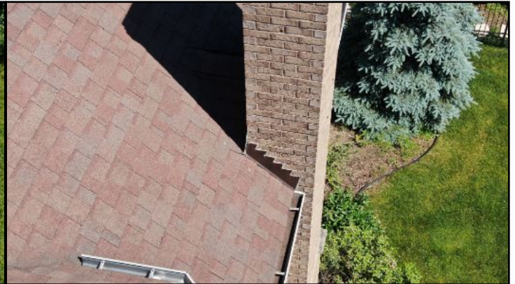
Flashing at base of chimney appears to be properly installed, no deficiencies noted.
