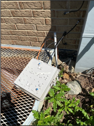
Cable boxes become disconnected from the house recommend repair
