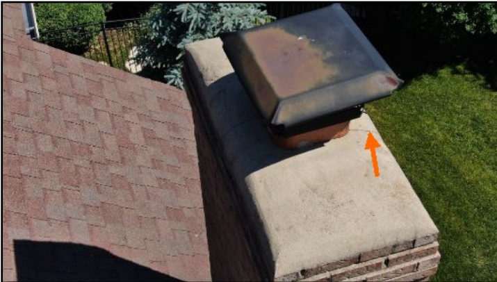
Masonry chimney cap is cracked
