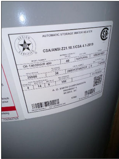
Water Heater Data Plate
