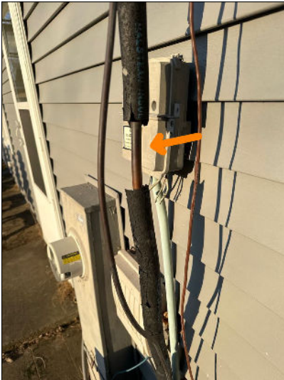
Missing insulation
