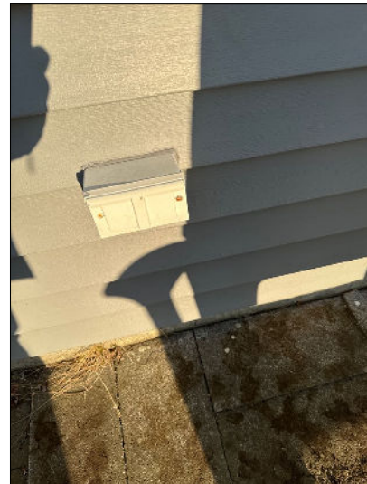
GFCI Outlet at - Rear did not trip when tested.
