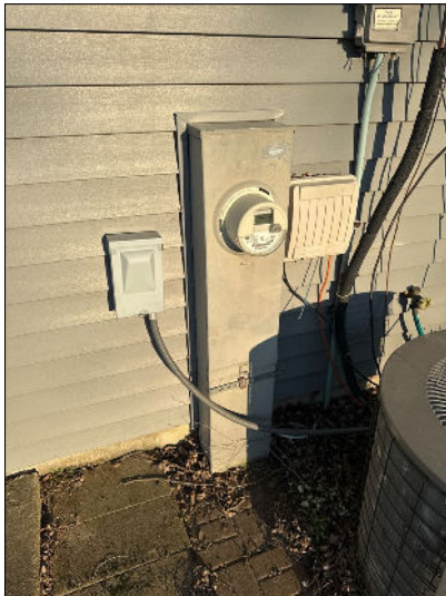
Underground Electric Service
