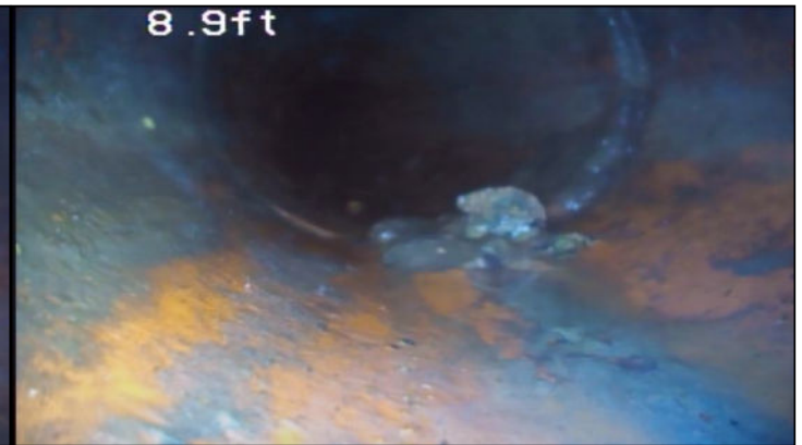
Deposits/Material buildup noted which are affecting the drainage flow.
