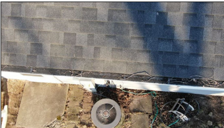
Gutters need to be cleaned.
