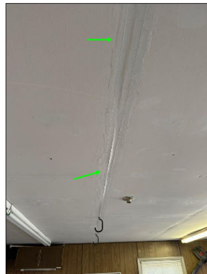
Failing drywall tape
