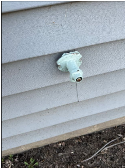
Missing / Broken handle noted at the time of the inspection on Front
