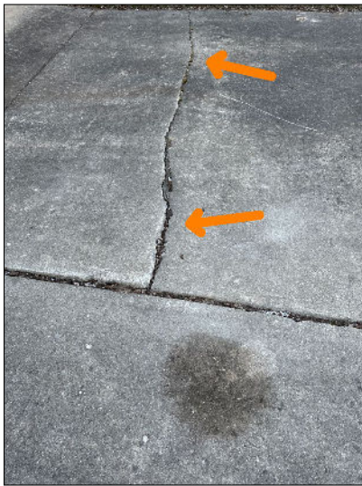
Potential Trip Hazard(s) at driveway/sidewalk; monitor / repair as necessary
