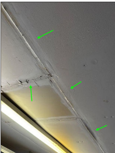
Failing drywall tape/patched area
