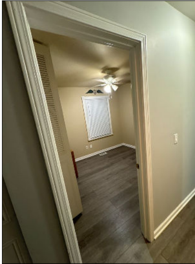
Door missing / NOT installed.
